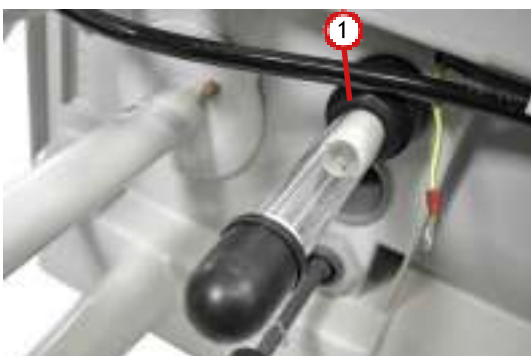
Fig. 8.1.2.6: UV lamp in quartz glass tube.
