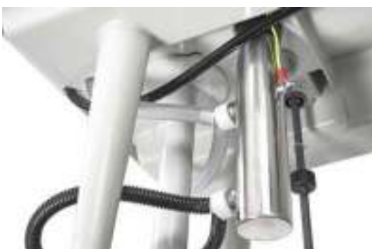
Fig. 8.1.2.8: UV disinfection unit, complete
