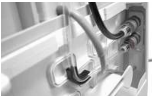
Fig. 7.4.1.10: Connection of power cable, if necessary AWS &
